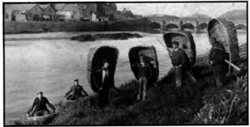
Photograph from the 1890's showing traditional Welsh coracle, built using ash lathes to form the basket, and covered in cowhide.
