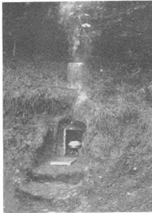
Camp Oven. Built in the side of a Bank.
