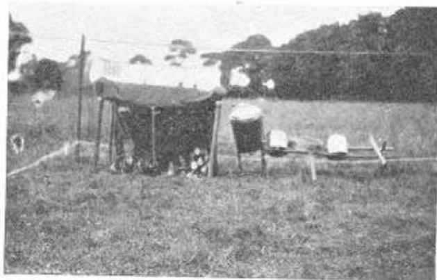
Wood Shelter and Dixie Rack.
