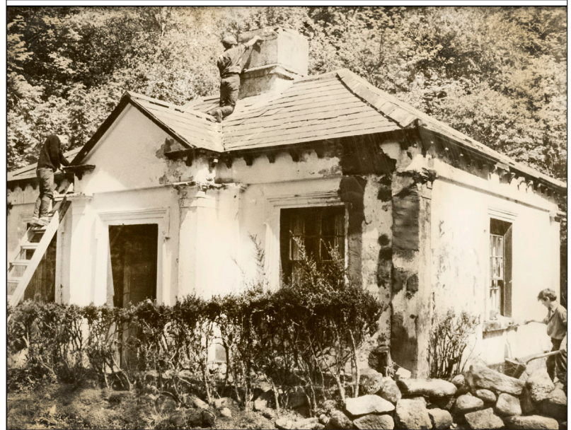
The Gate Lodge under repair in 1970's
