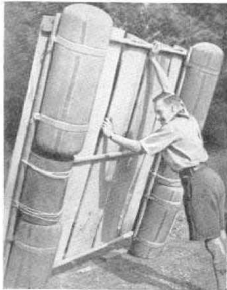
ALTERNATIVE METHOD OF ATTACHING INFLATED BUOYS
